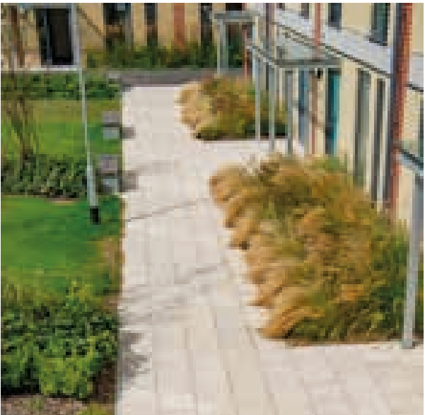
Permeable concrete paving slabs. Laid in diamond pattern.
